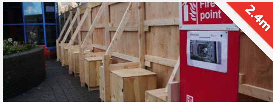
Free standing hoarding with 800kg ballast boxes.
