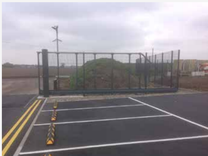
Automated Protek 1000 sliding gate.
