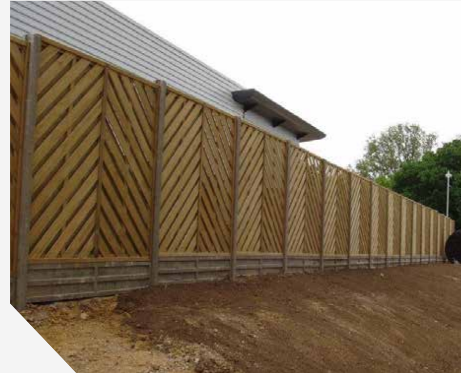
Concrete post and gravel boards with a PAR chevron panel.
