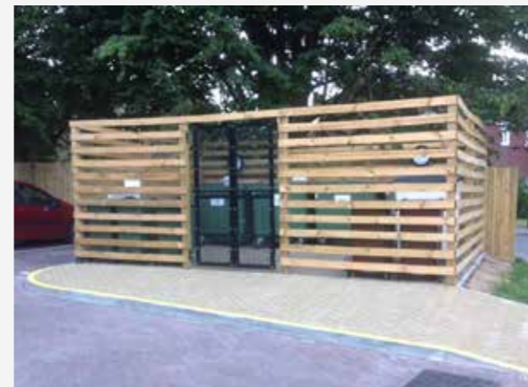
Hit and miss linear bin store on a dug in system.
